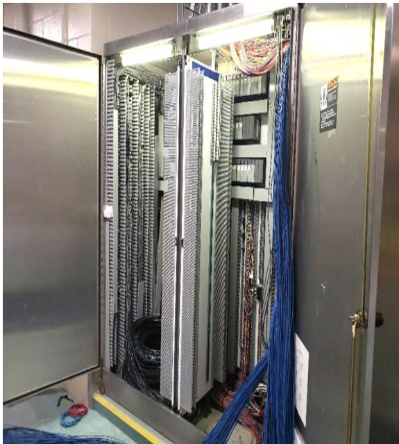
New Backplane Sub-Panel in Existing Control Panels
