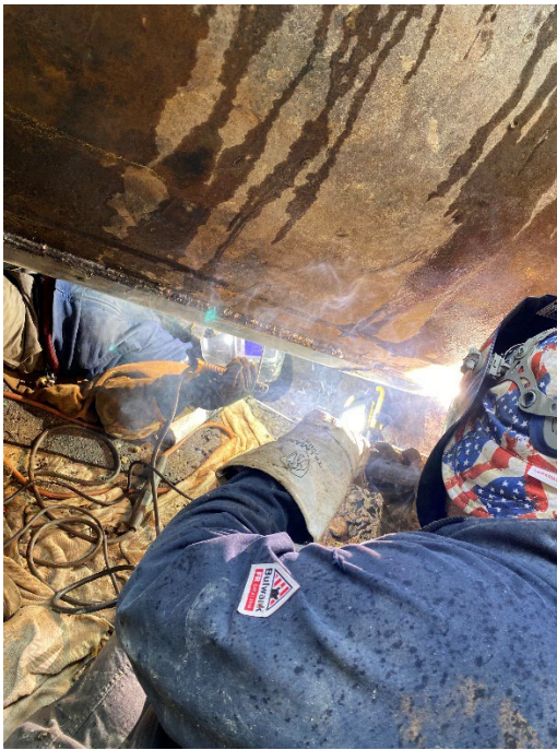
Figure 6 – Welding Rolled Steel Plates
