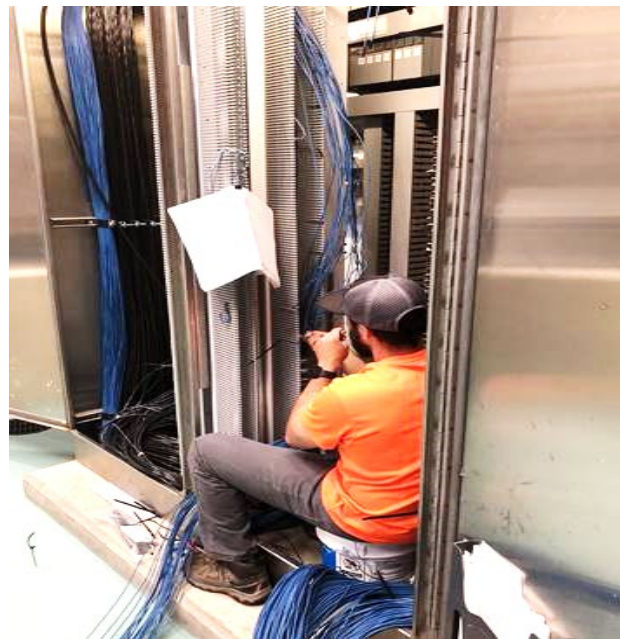
Terminating Control Wires on New Backplane Sub-Panel
