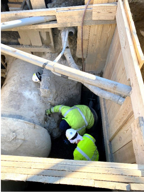
Figure 4 – Concrete Removal
