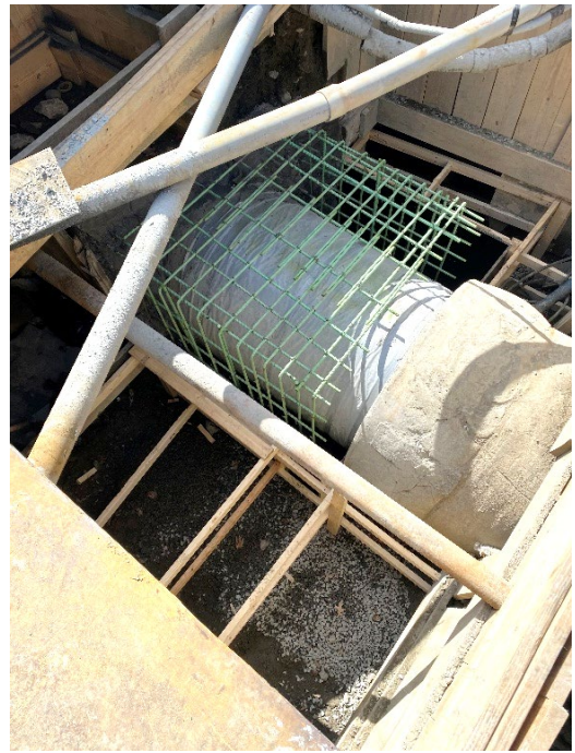
Figure 7 – Rebar and Concrete Installation
